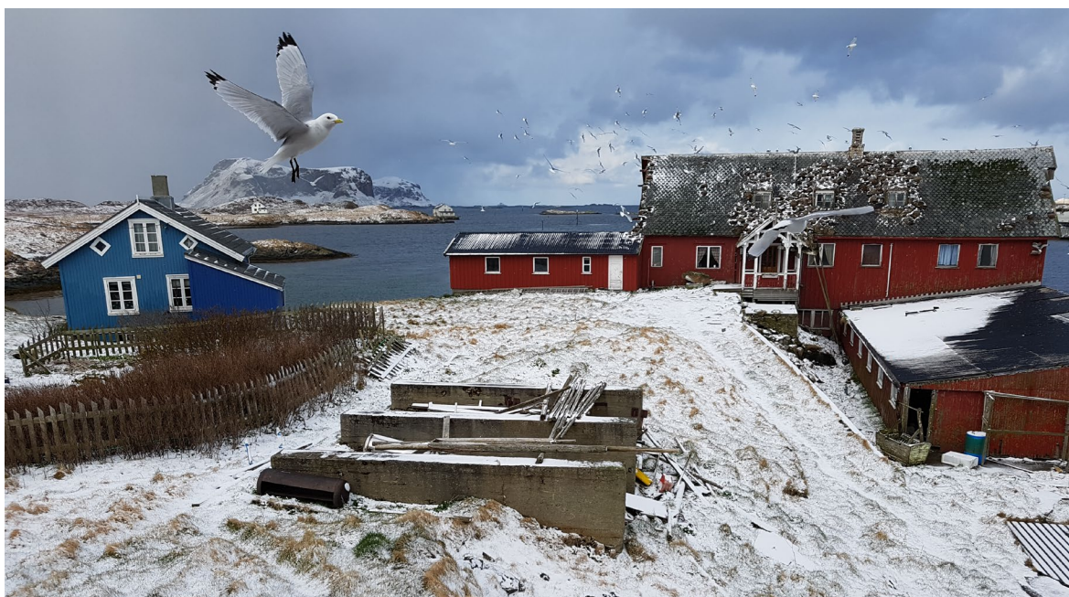
Figure S2. View of Nilssenuset and the construction site on Kårøya on 13 May 2020. The Kittiwake hotel was built on the concrete walls in the foreground, which supported two large fuel tanks in the 1930s. The island in the background is the 205 m high Vedø, four km southwest of the harbour, which supported the large cliff-breeding population that became extinct in 2020. © Tycho Anker-Nilssen.
