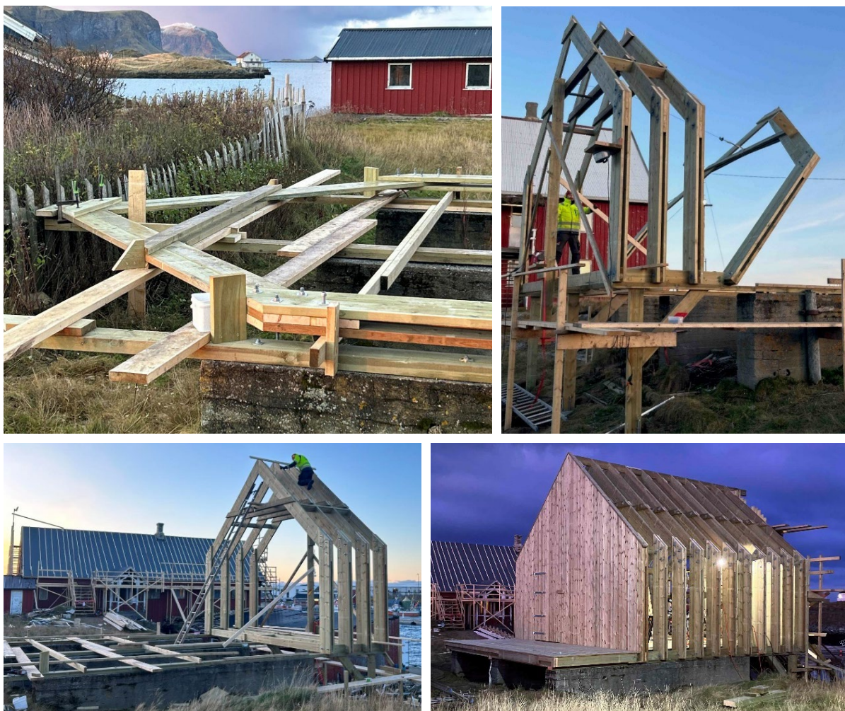
Figure S6. Connecting supporting beams and raising the structural envelope of the Kittiwake hotel in October–November 2023, alongside repairs to the roof of Nilssenhuset (seen in the background on the lower panels) was also repaired. All framework was built using pressure-treated timber. © DSN Entreprenør AS, Svolvær.
