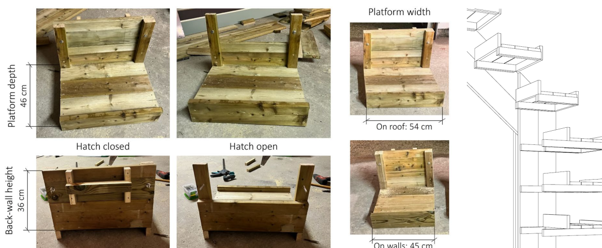
Figure S7. In January 2024, the 210 nest platforms were constructed from 28 \times 120 mm pressure-treated decking planks and prefabricated indoors using stainless steel decking screws prior to being fitted onto the structural envelope (right, see also Figures S8–S9). To allow easy access for measuring eggs and chicks, the removable upper half of the back wall was attached using two stainless steel machine screws and wing nuts.
